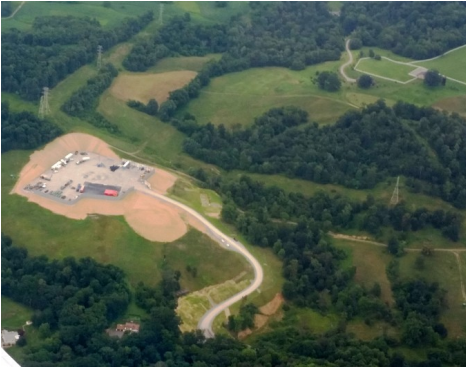
The ‘Gulick’ well pad, seen from above Deer Lakes Park.
